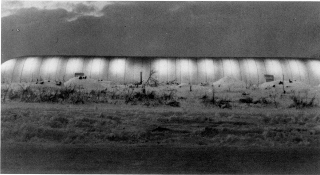
Top: The erection of the bubble of this air-supported structure for Computer Technology took about an hour and the entire construction sequence a few weeks.
